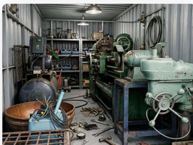
Inside Mobile Machineries No.1
